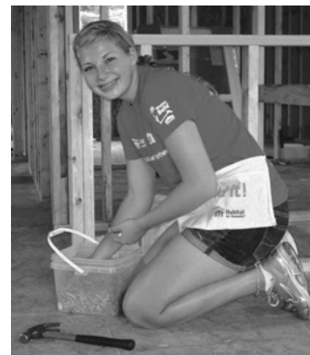
Madeson working at our 2 nd Women Build Day this year!
